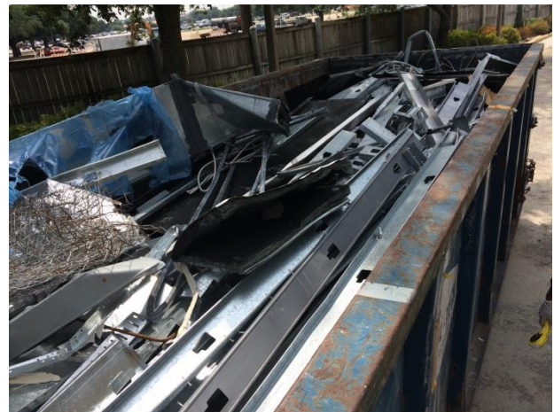
Figure 1. Renovation debris in the dumpster.
